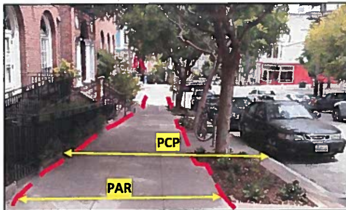
Figure 1: PAR within Pedestrian Circulation Path
