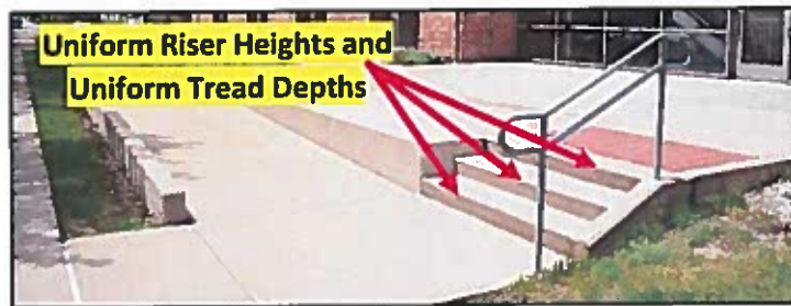
Figure 109: Uniform Riser Height and Tread Depth
