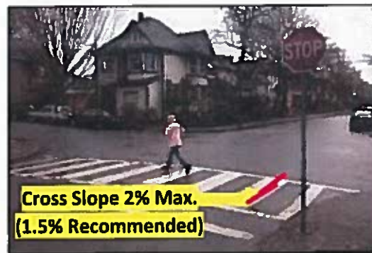
Figure 12: Pedestrian Street Crossing with Stop Control
