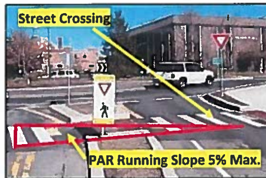
Figure 10: PAR Running Slope within Street Crossings
