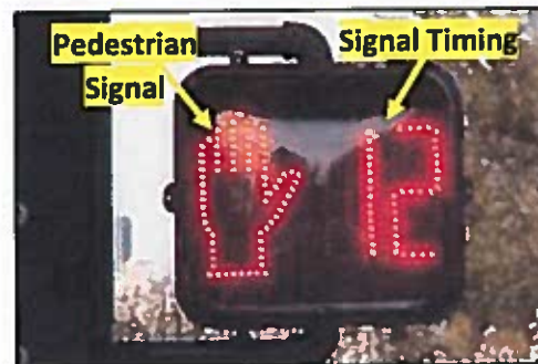
Figure 78: Pedestrian Signals Combined with Pedestrian Signal Timing
