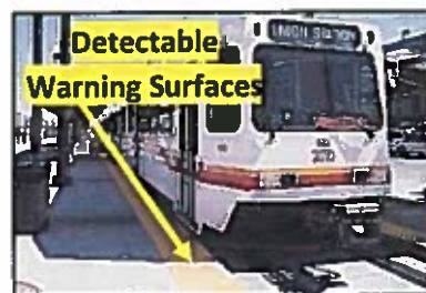
Figure 59: DWS at Boarding and Alighting Areas
