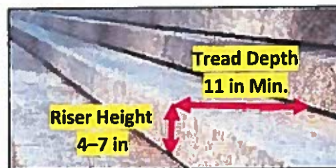
Figure 110: Riser and Tread Dimensions
