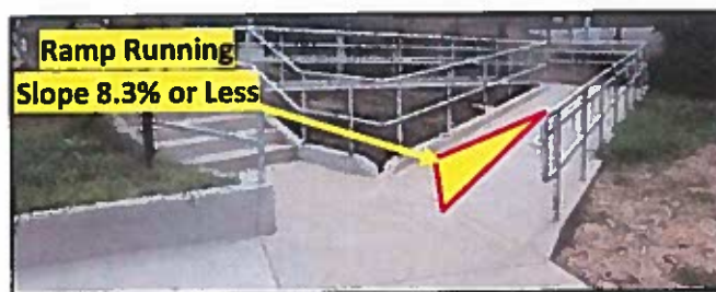
Figure 104: Ramp Running Slope
