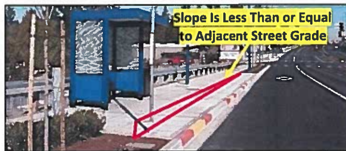
Figure 86: Slope of Boarding and Alighting—Parallel to Street
