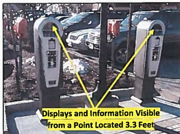
Figure 94: Visibility Requirement for Displays at Parking Pay Stations
