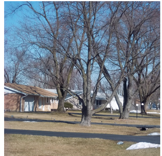
Fernway Single Family Home, Orland Park
