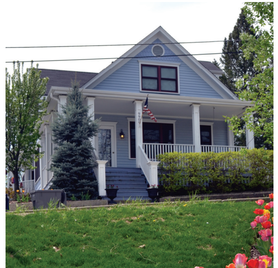
Old Orland Single Family Home, Orland Park
