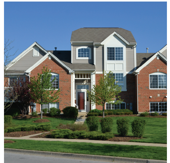
Orland Crossing Townhomes, Orland Park
