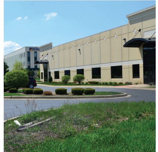
Orland Park Business Center, Orland Park
