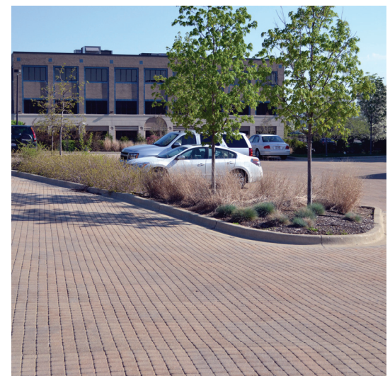
Porous Paving, John Humphrey Drive Offices, Orland Park
