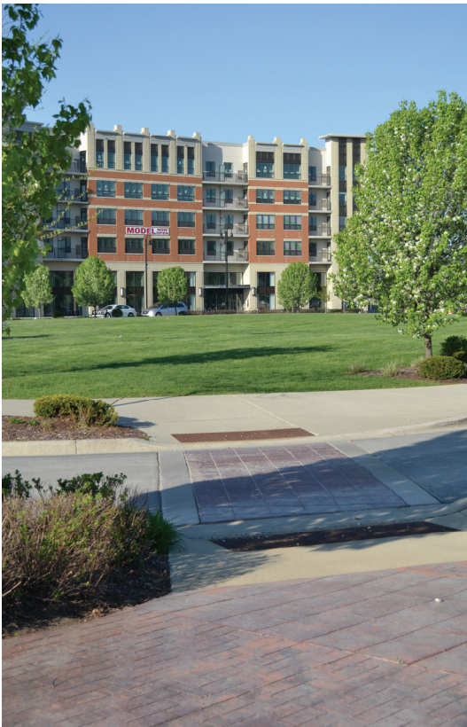
Ninety7Fifty on the Park and Crescent Park, Orland Park
