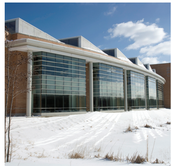
Orland Park Public Library, Orland Park. (Wehmeier, 2013)
