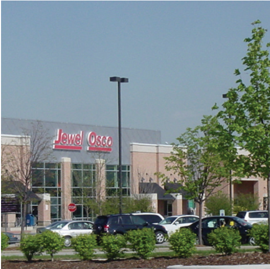
Jewel at Marley Creek Crossing, Orland Park
