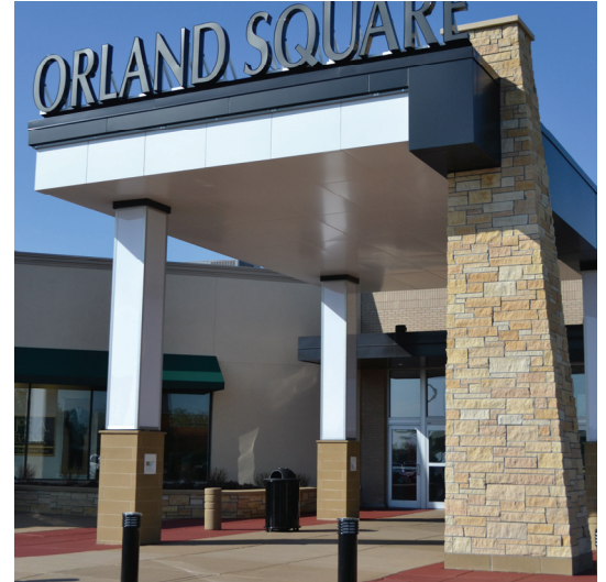
Orland Square Mall, Orland Park
