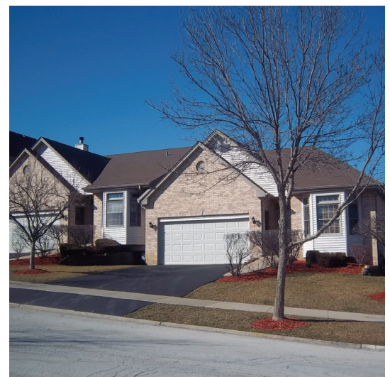
Fernway Townhome, Orland Park
