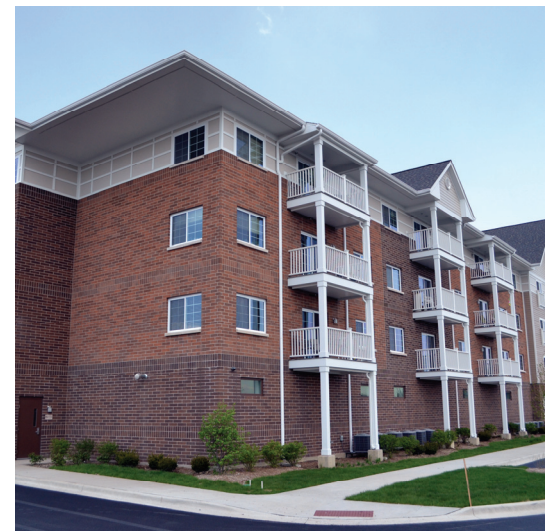
Thomas Place Senior Living Facility, Orland Park
