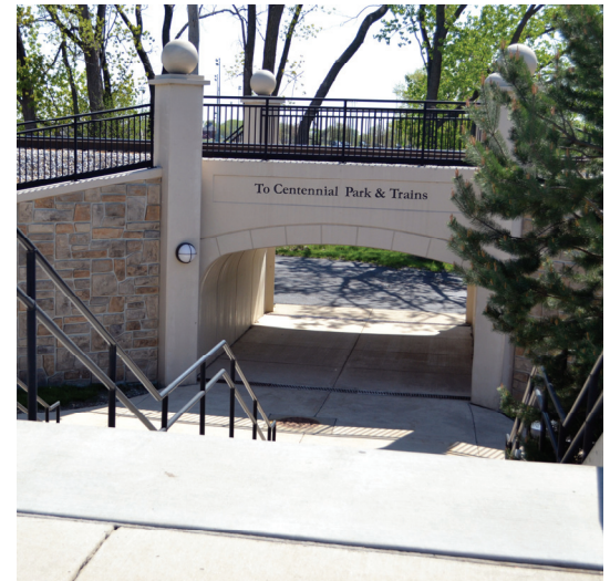
153rd Metra/Centennial Park Pedestrian Tunnel, Orland Park
