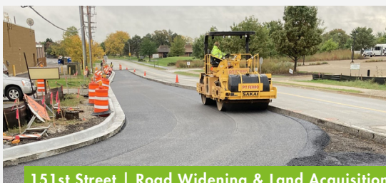
151st Street | Road Widening & Land Acquisition
