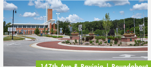
147th Ave & Ravinia | Roundabout
