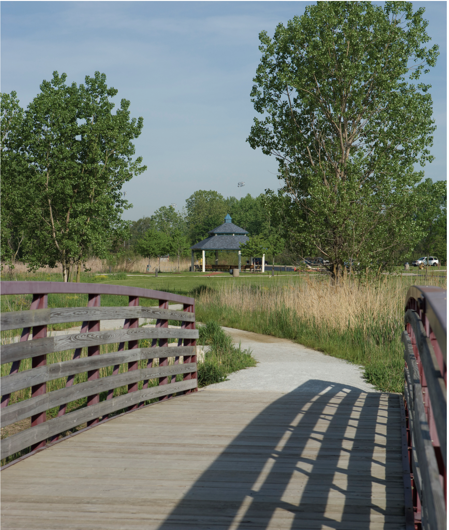
Multi-Use Path Crossing, Orland Park. (Wehmeier, 2013)
