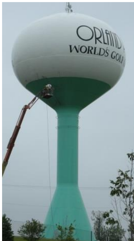
Existing Condition of Water Tower #8
