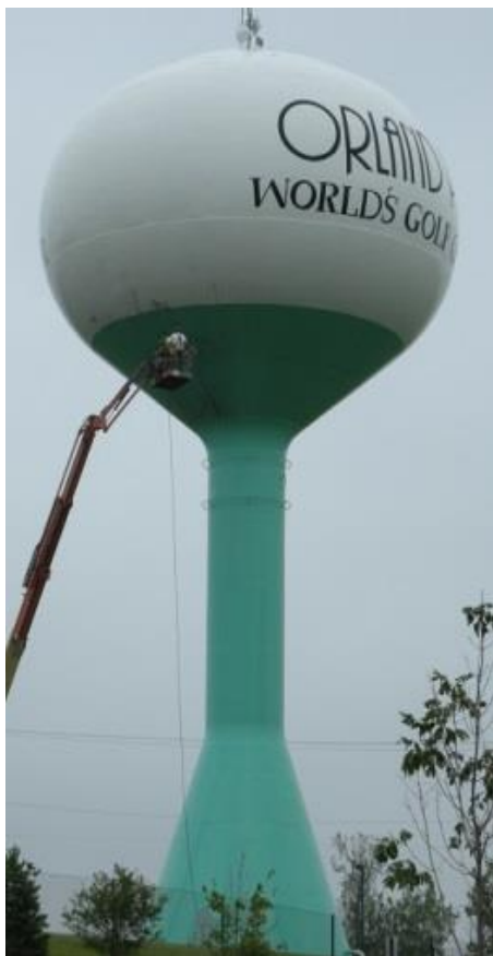
Existing Condition of Water Tower
