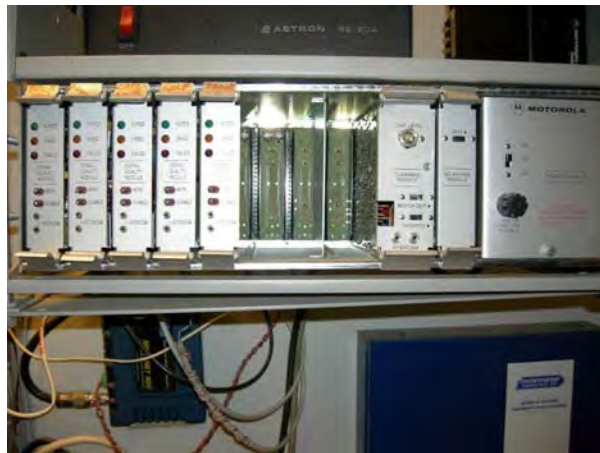
Voter chassis with voter modules and power supply
