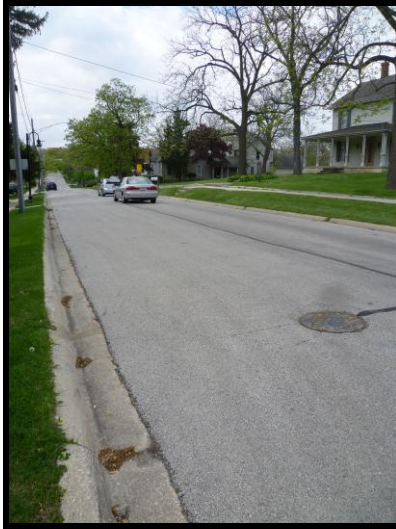
VIEW WEST ALONG 144 TH PLACE
