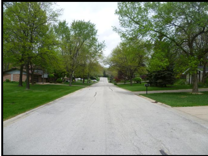
VIEW NORTH ALONG WESTWOOD DRIVE
