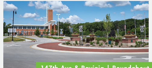
147th Ave & Ravinia | Roundabout
