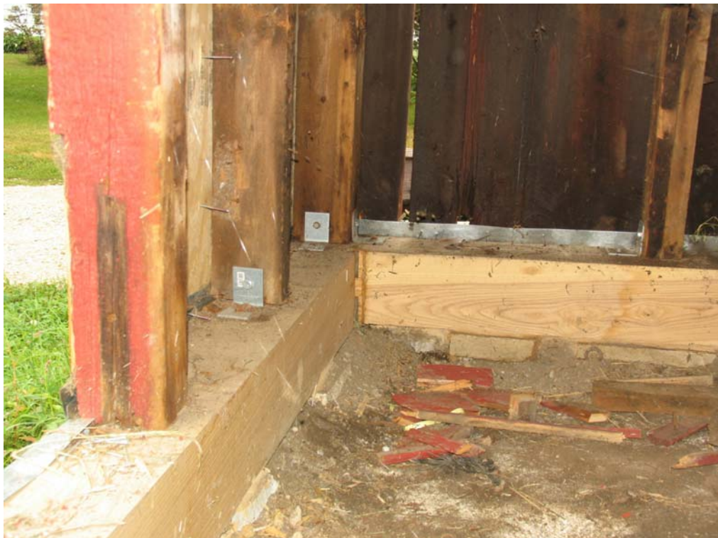
Interior of new construction on northwest corner of barn.
