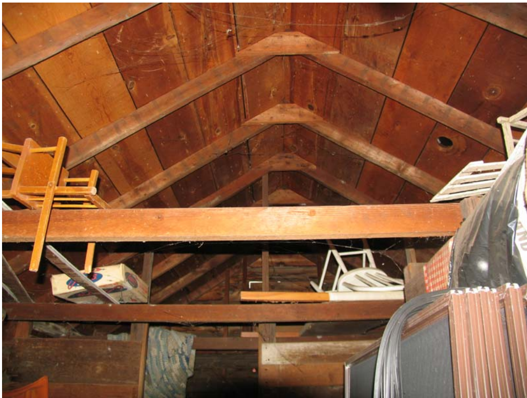
View to east. Ceiling of Shed 3.
