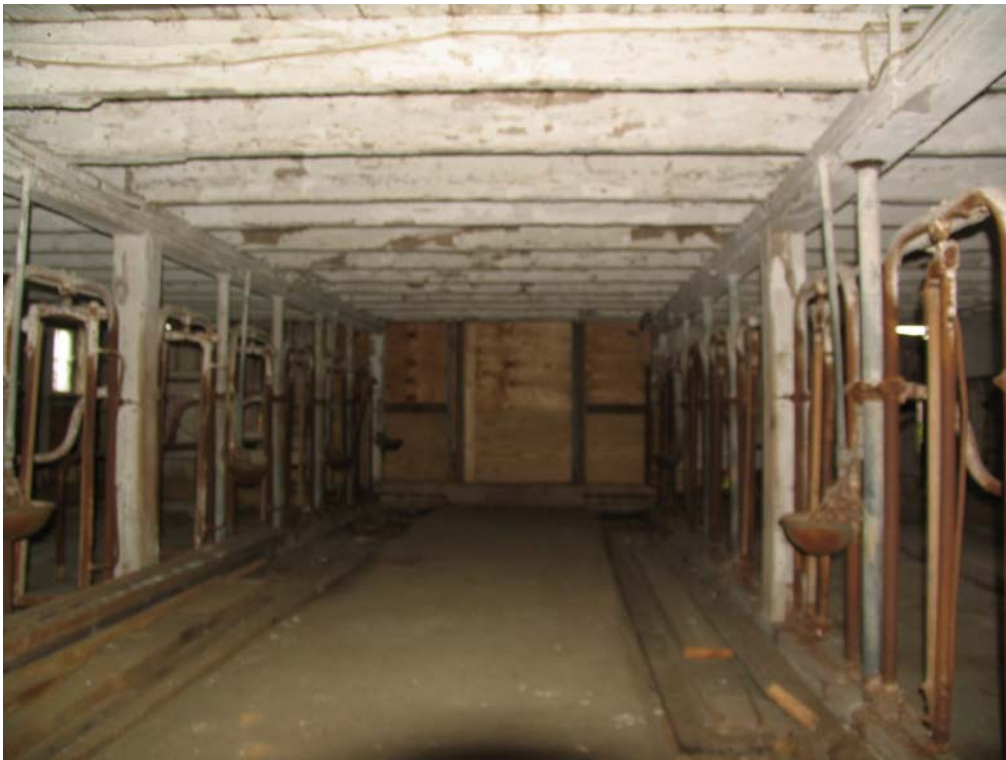
View to south. South end, main floor of barn.
