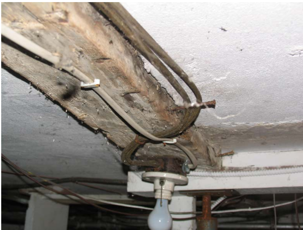
Basement ceiling beam.
