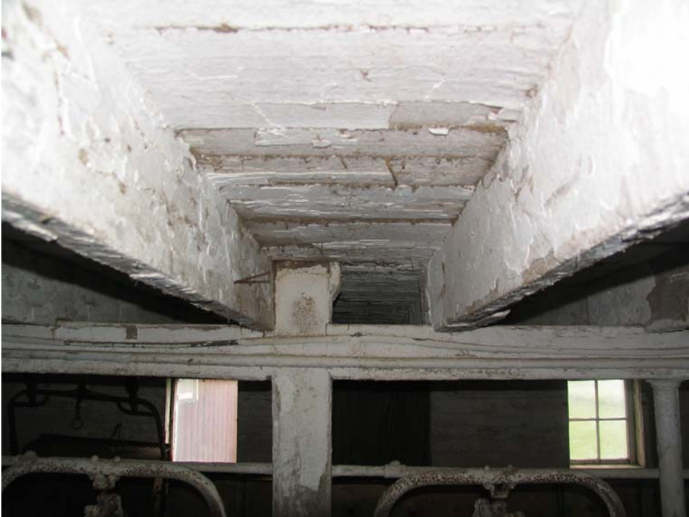
Close-up view of ceiling in south end of barn.
