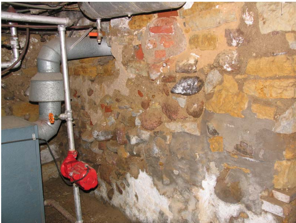
View to southwest. Close-up view of interior basement wall.
