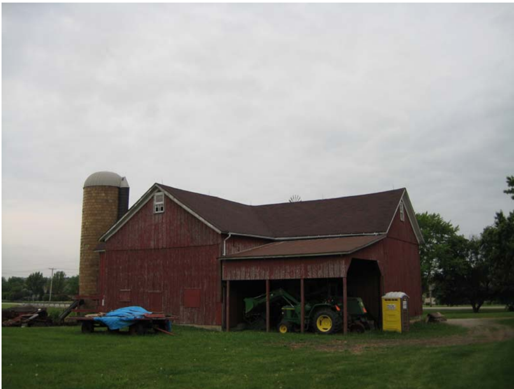
View to west. East elevation of Barn at 11CK1060.
