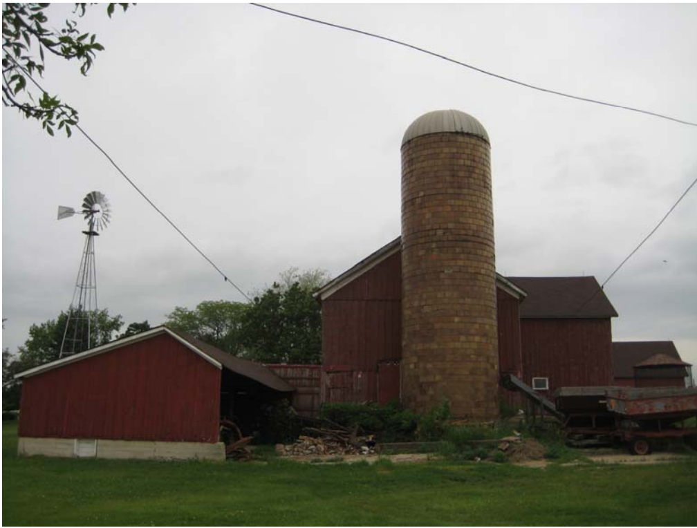
View to north. South elevation of Barn and Tile Silo at 11CK1060.
