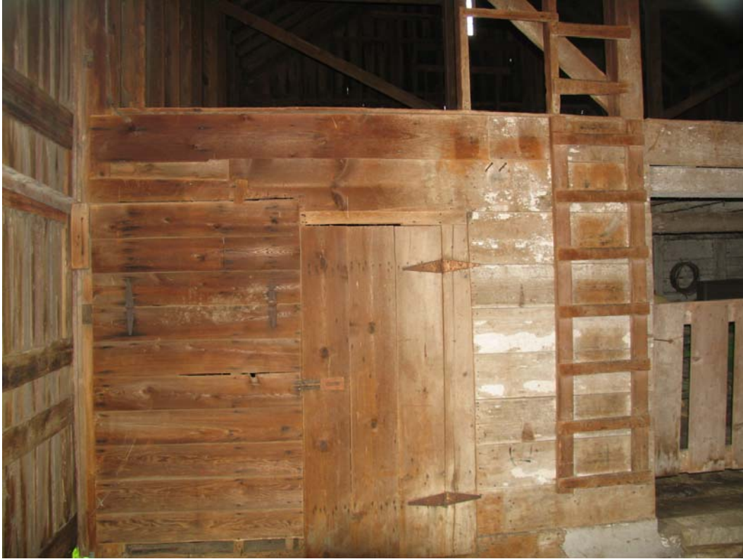
View to North. North end of barn.
