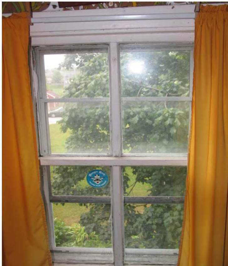
View to south. Close-up of window in upstairs bedroom 1.
