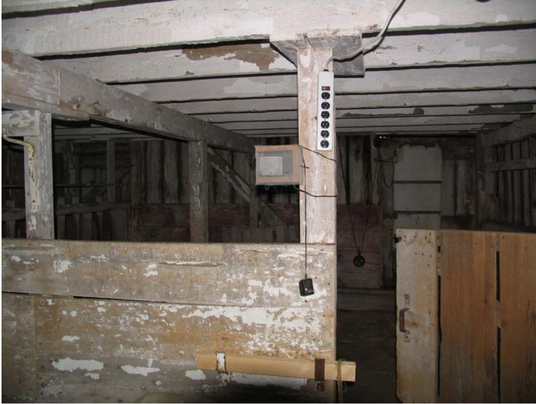
View to east. East end of barn.
