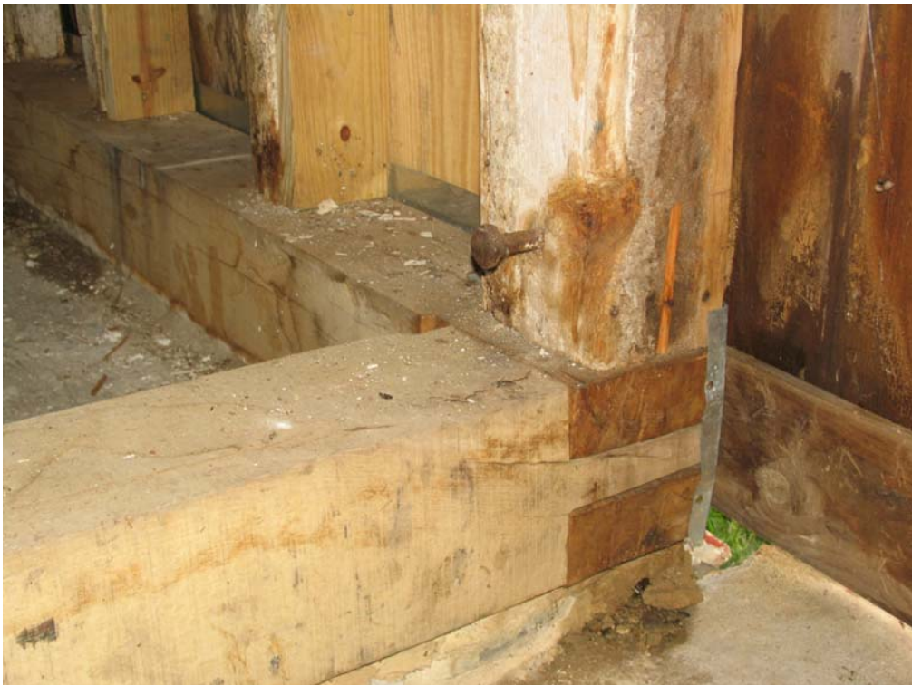
Close-up view of modern bracing and leveling work on the barn.
