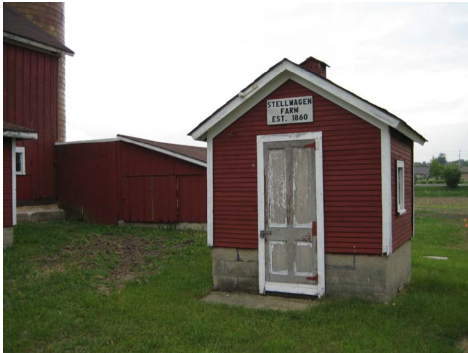
View to south. North elevation of Pump House at 11CK1060.
