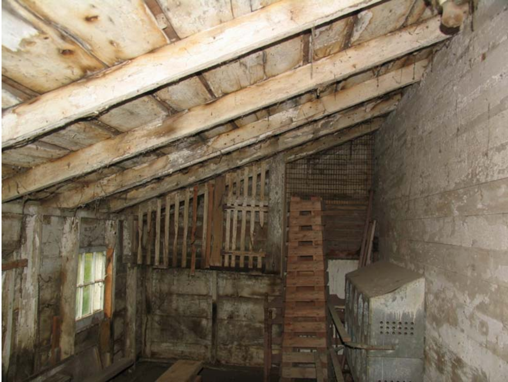
View to west. Interior of chicken coop at Shed 2.
