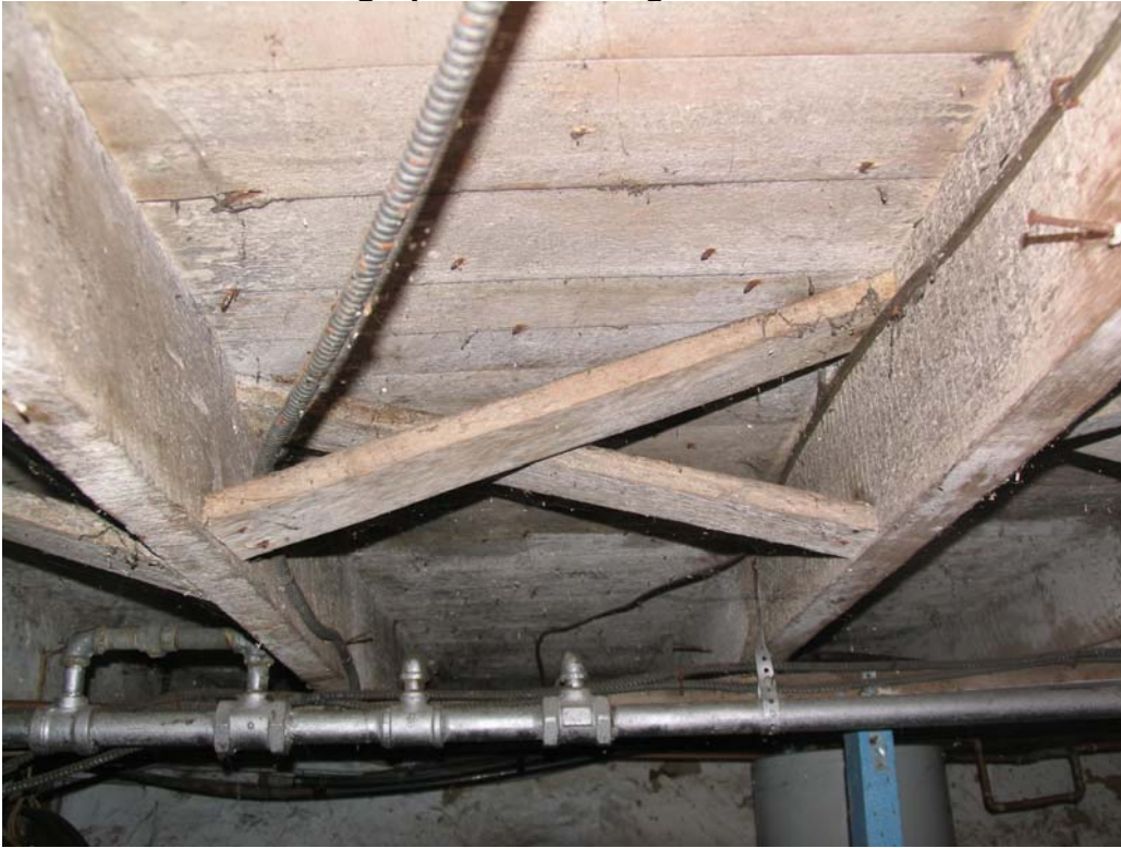
Close-up view of basement ceiling.
