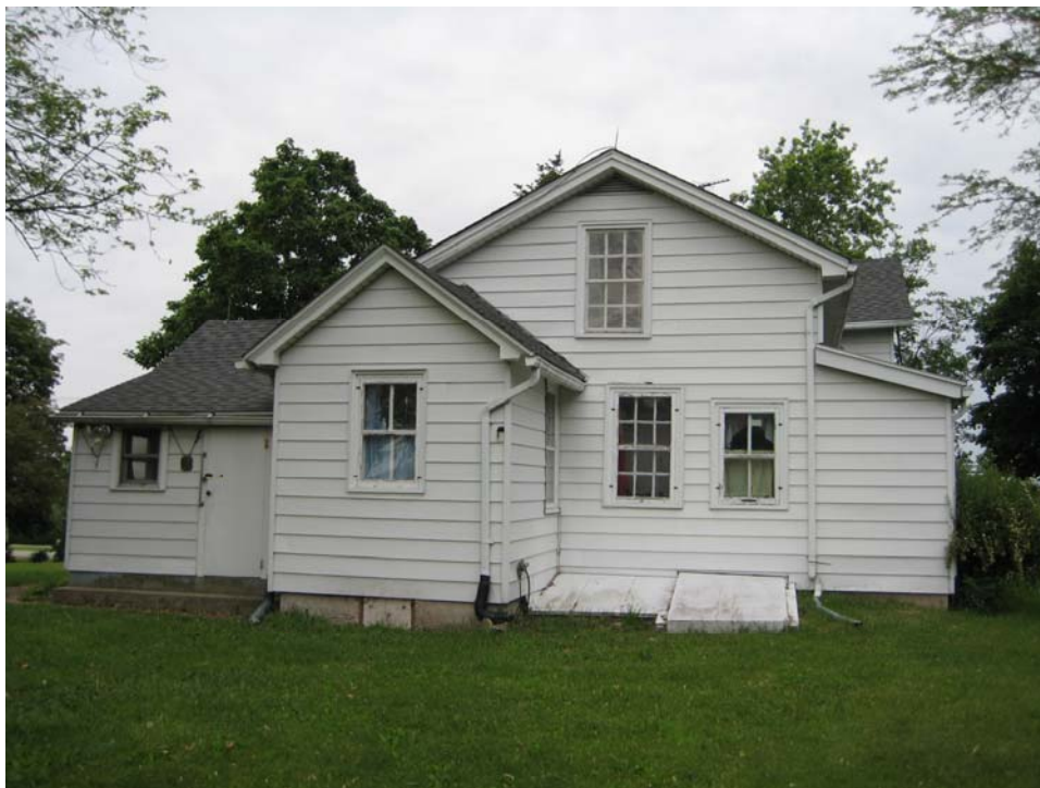
View to west. East elevation of Residence at 11CK1060.
