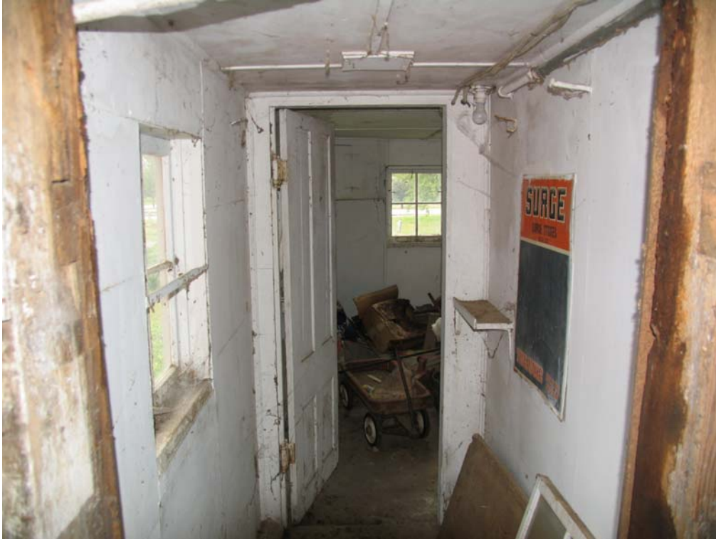
View to east. Milk house attached to barn.
