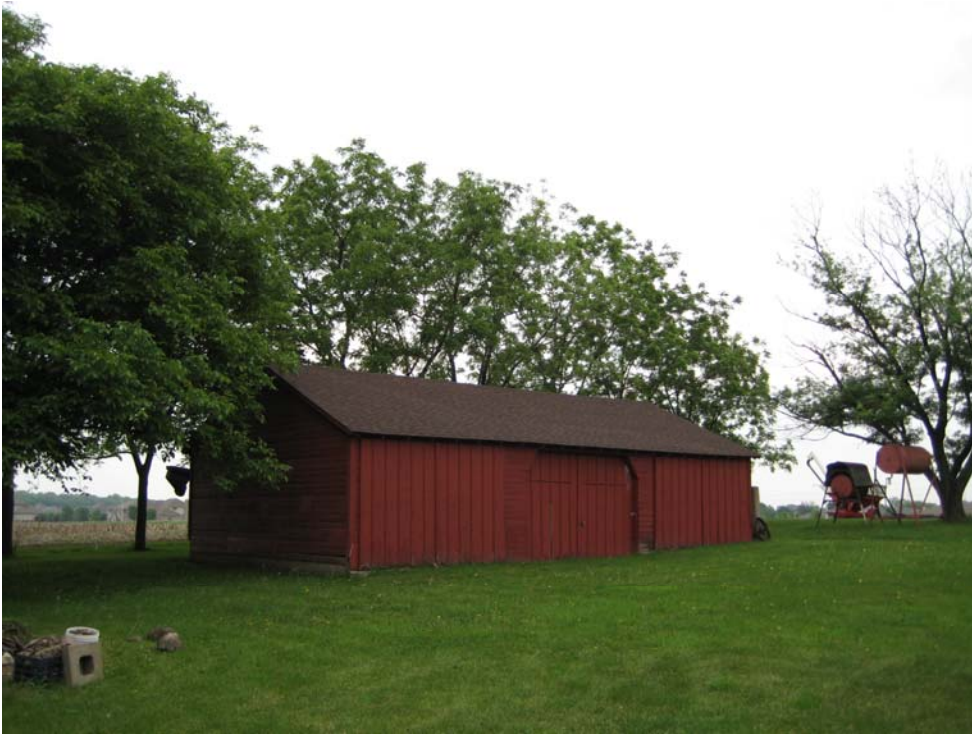
View to east. West elevation of Equipment Shed at 11CK1060.
