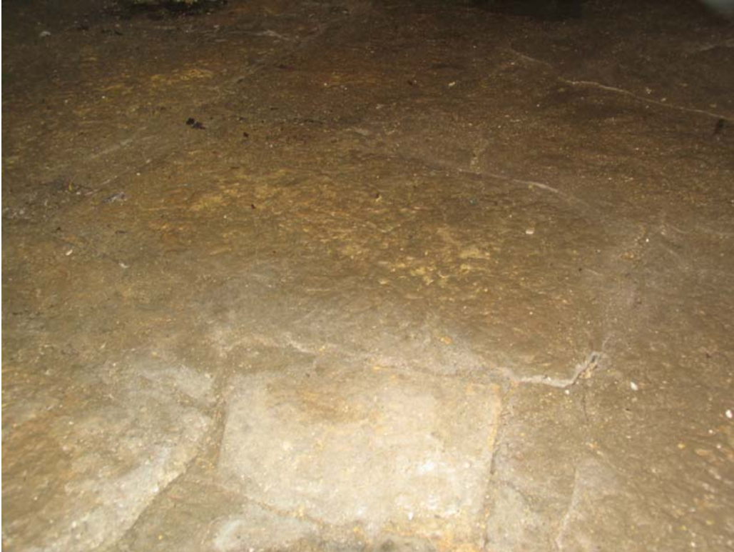
Representative view of basement floor.
