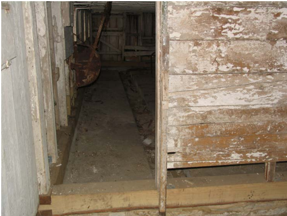
Modern construction/repair in barn.
