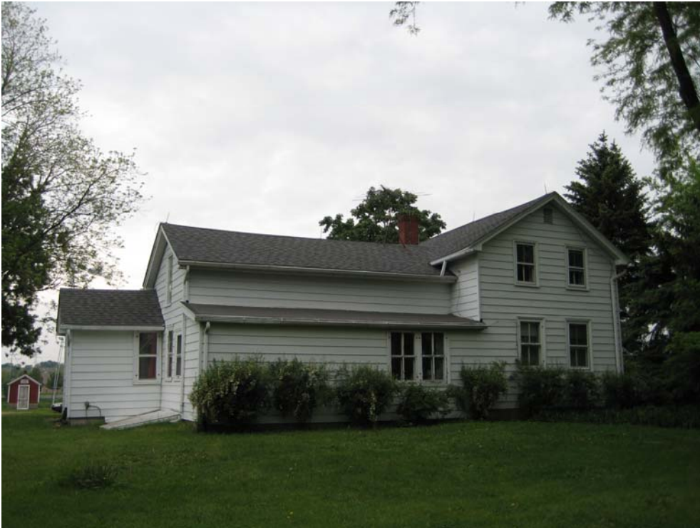
View to south. North elevation of Residence at 11CK1060.
