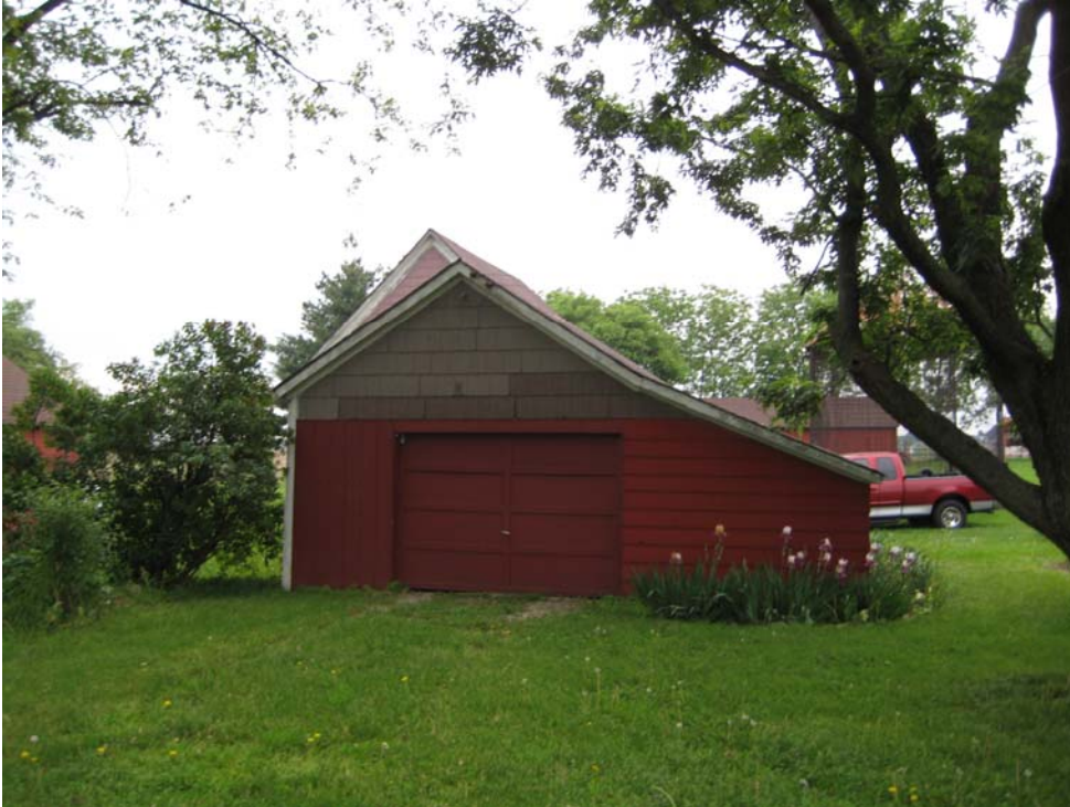
View to east. West elevation of shed 2 at 11CK1060.
