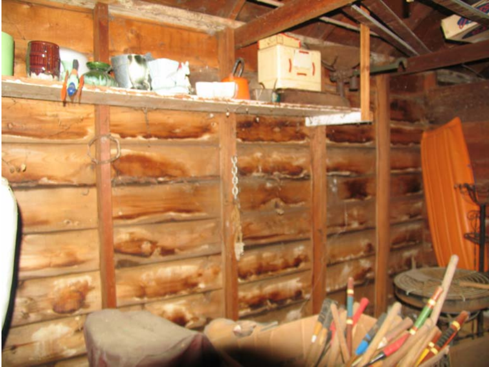
North interior elevation of Shed 3.
