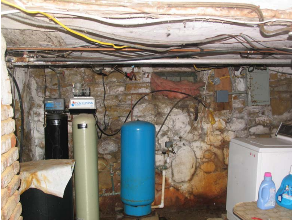
View to south. South elevation of basement wall.
