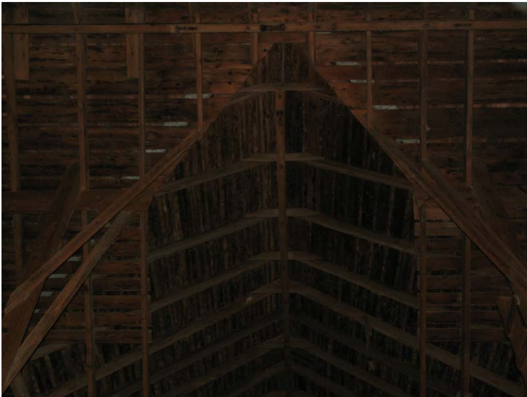
Representative view of barn ceiling.
