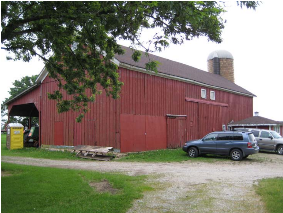
View to southeast. North and west elevation of Barn at 11CK1060.
